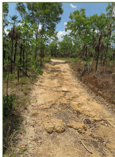
Figure 6: The track running in and out of the Meade Road reserve makes fencing the northern boundary problematic (in addition to the fact that the river crosses the boundary).
