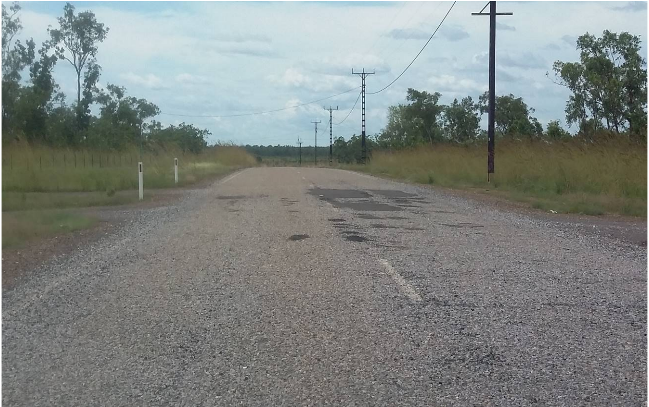
Figure 3 - Sealed road requiring renewal
