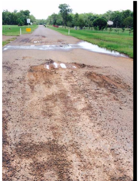
Bundey Road Damage Picture 1
