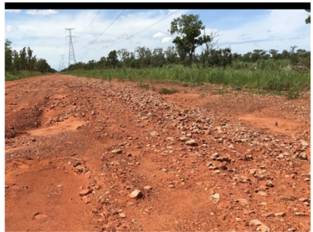
Brougham Road Damage Picture 2
