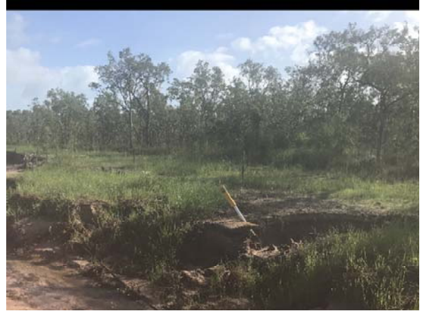
Trippe Road North Damage Picture 2
