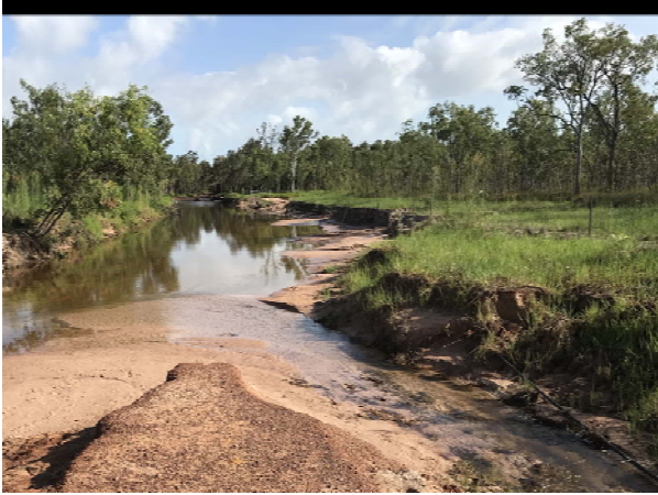
Trippe Road North Damage Picture 1
