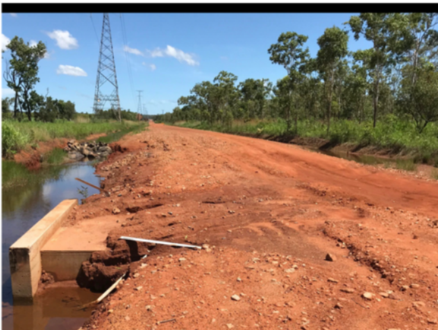
Brougham Road Damage Picture 1
