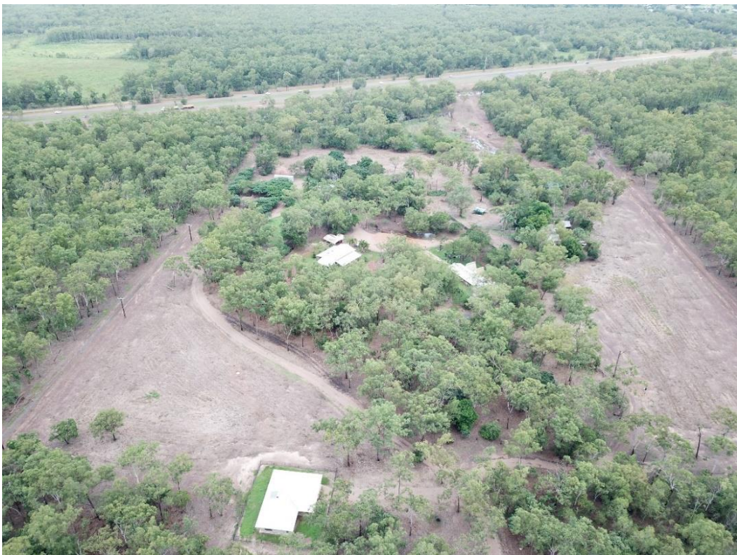
Photograph 3 – Sites existing buildings
