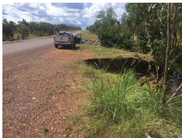
Finn Road Damage Picture 2
