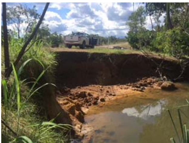
Finn Road Damage Picture 1
